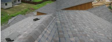
The roof is composition shingle and appears to be functioning as intended.
