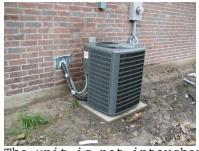
The unit is not interchanging the air properly, between the return air and outlet air.(9 degrees) Barz Inspections recommends having the HVAC contractor evaluate and repair this issue.
