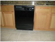
The dishwasher was loose in the cabinet hole and should be firmly attached. Functioned properly on the day of the inspection.
