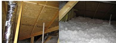
The roof and attic appeared to be functioning as intended on the day of the inspection. There appears to be approximately 8-12 inches of insulation in most locations of the attic.
