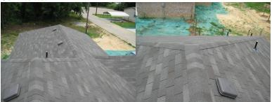
The roof is composition shingle and appears to be functioning as intended.
