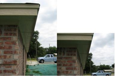
The home has no soffit vents along the front of the home and only one on the right side. This is inadequate attic ventilation for this home and more vents need to be added.
