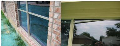
The window screens have not been installed as of the time of the inspection. One of the front windows has a piece of the plastic strips that is loose and needs to be reattached. The plastic strips are what hold the glass in place.
